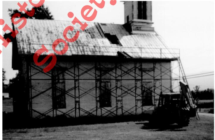
The long process of restoring the Heritage Center began shortly after its purchase in 1988. Here, scaffolding has been erected and a pay-loader has been brought in to lift lumber to the roof so that volunteer workmen can repair some lumber in the steeple that was destroyed by carpenter ants and to fix a six inch sag in the roof. Inside, a buttress was also built to shore up beams while repairs were under way.
