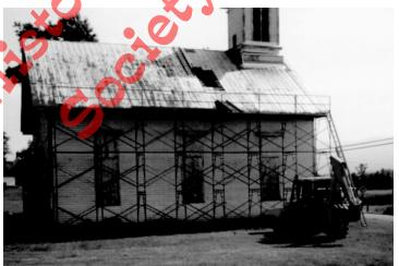
The long process of restoring the Heritage Center began shortly after its purchase in 1988. Here, scaffolding has been erected and a pay-loader has been brought in to lift lumber to the roof so that volunteer workmen can repair some lumber in the steeple that was destroyed by carpenter ants and to fix a six inch sag in the roof. Inside, a buttress was also built to shore up beams while repairs were under way.
